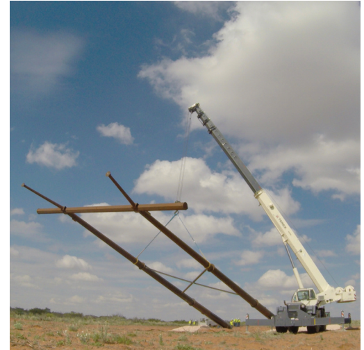
Crews set a structure about 25 miles west of Jal, New Mexico.
