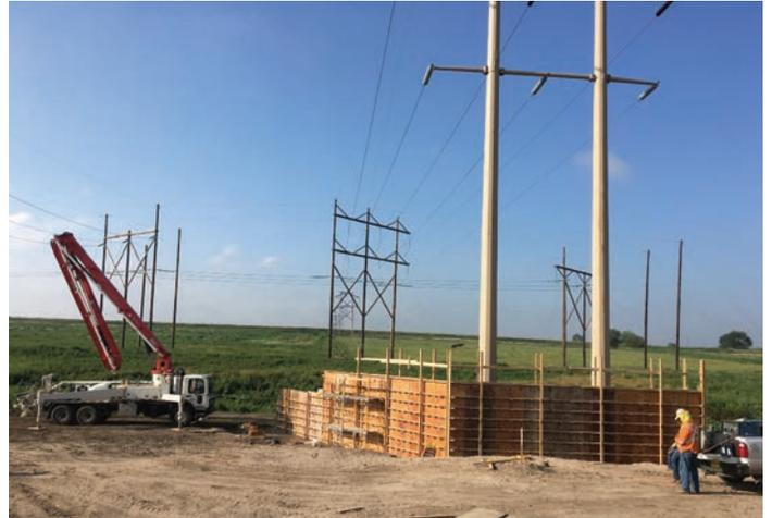
**Crews work on building a retaining wall in preparation for upgrades being made at Deaf Smith Substation in Hereford, Texas.**
